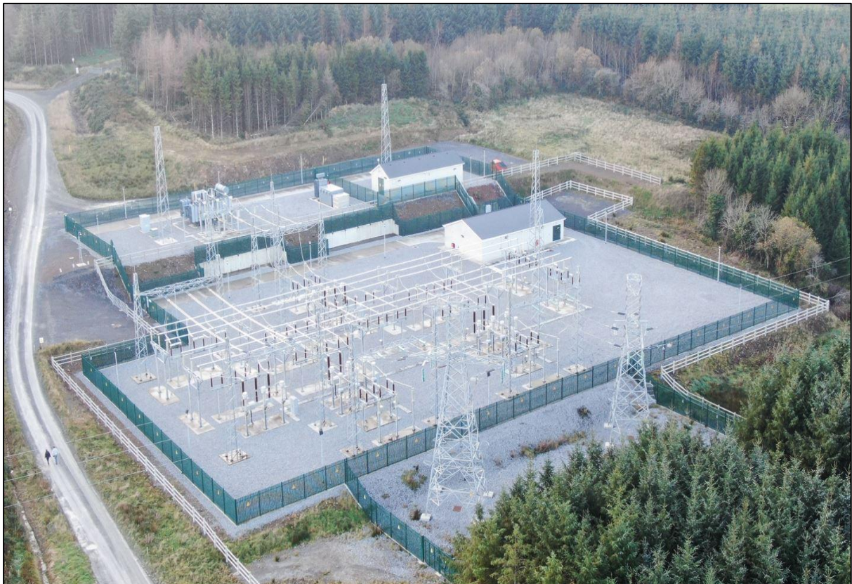
Figure 3: Typical 110kV AIS Substation
